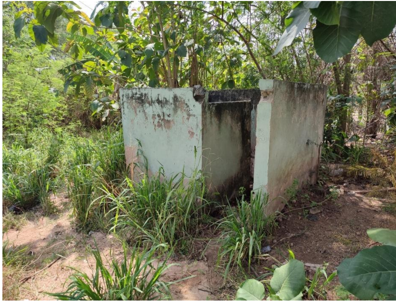
Figure 2. Example of existing washroom facilities in Kumasi, Ghana [site visit, 2023]
