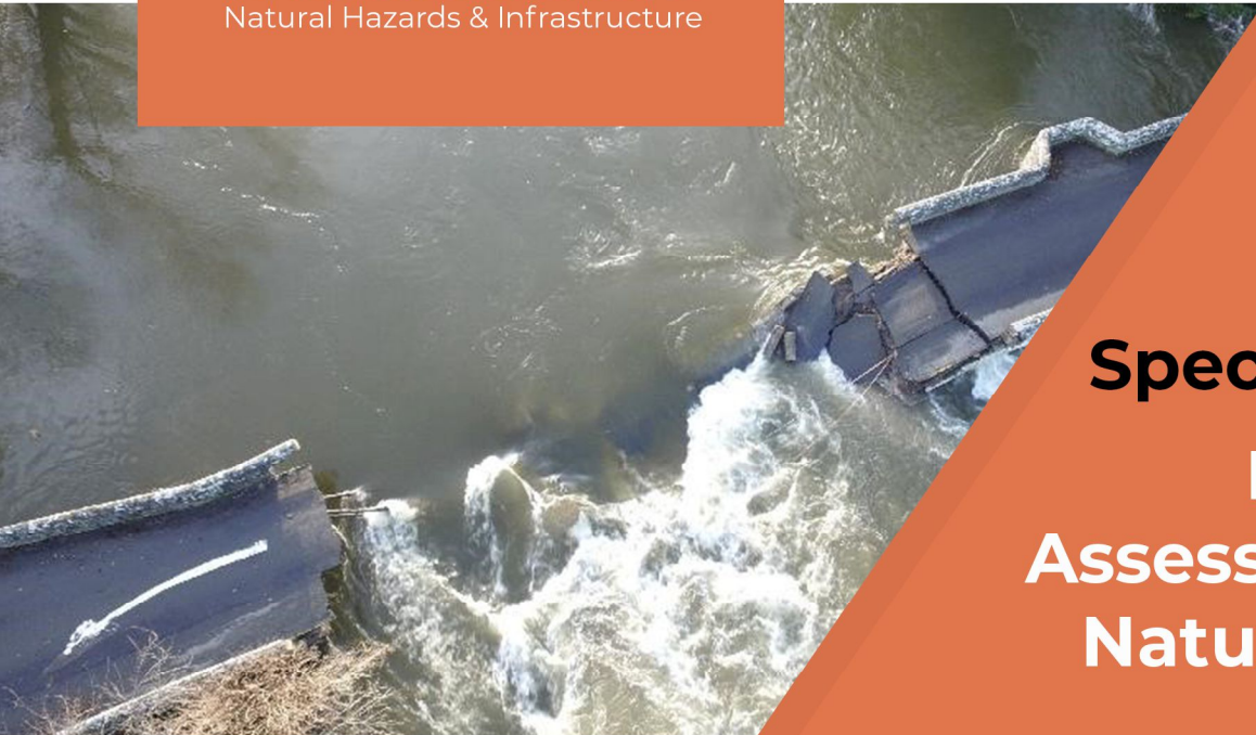
Aerial view of the collapsed Pooley Bridge in the aftermath of Cumbria Rainfalls in UK
